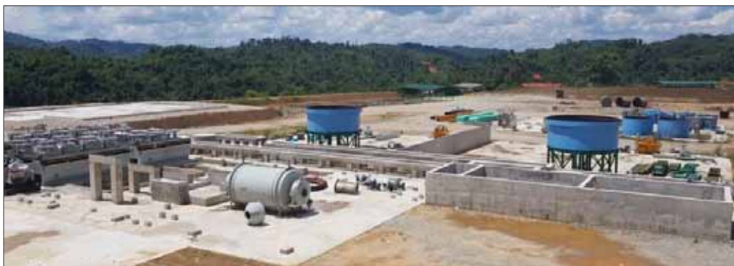
Figure 3.3 Construction of Sokor flotation plant – October 2019
