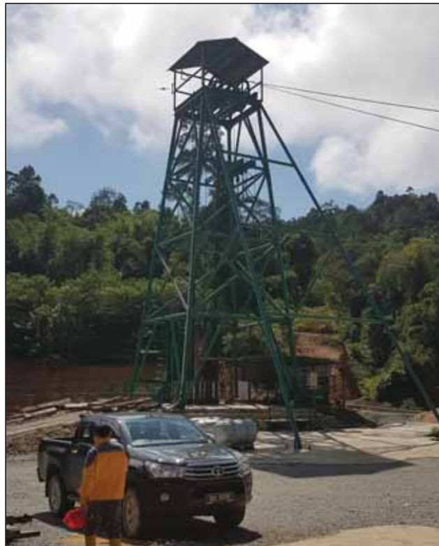
Figure 3.4 Ketubong shaft headframe – October 2019
