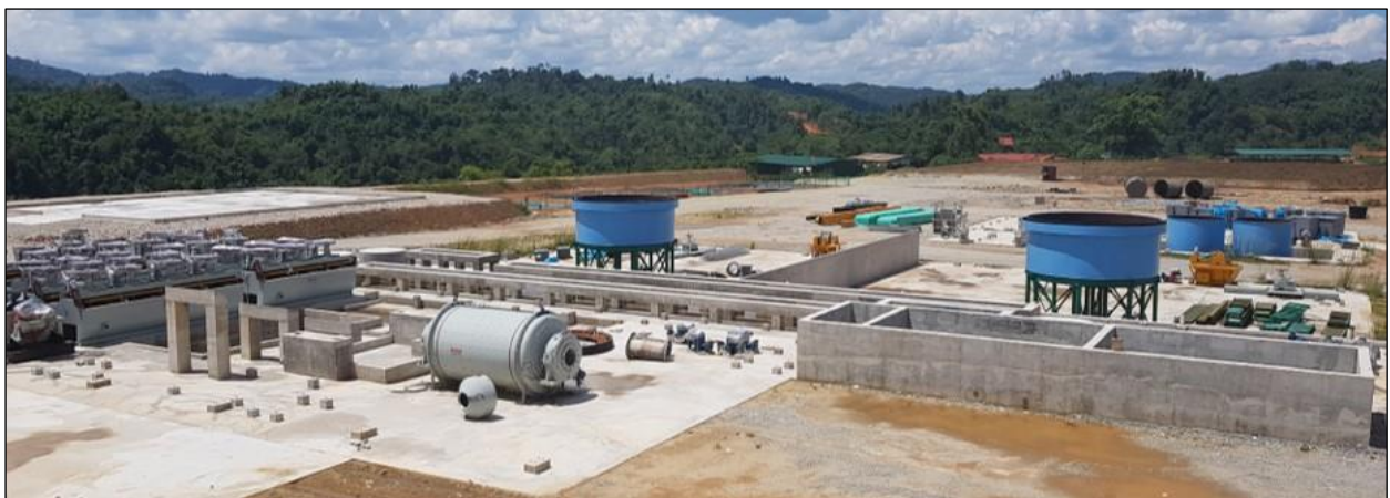
Figure 3.3 Construction of Sokor flotation plant – October 2019
