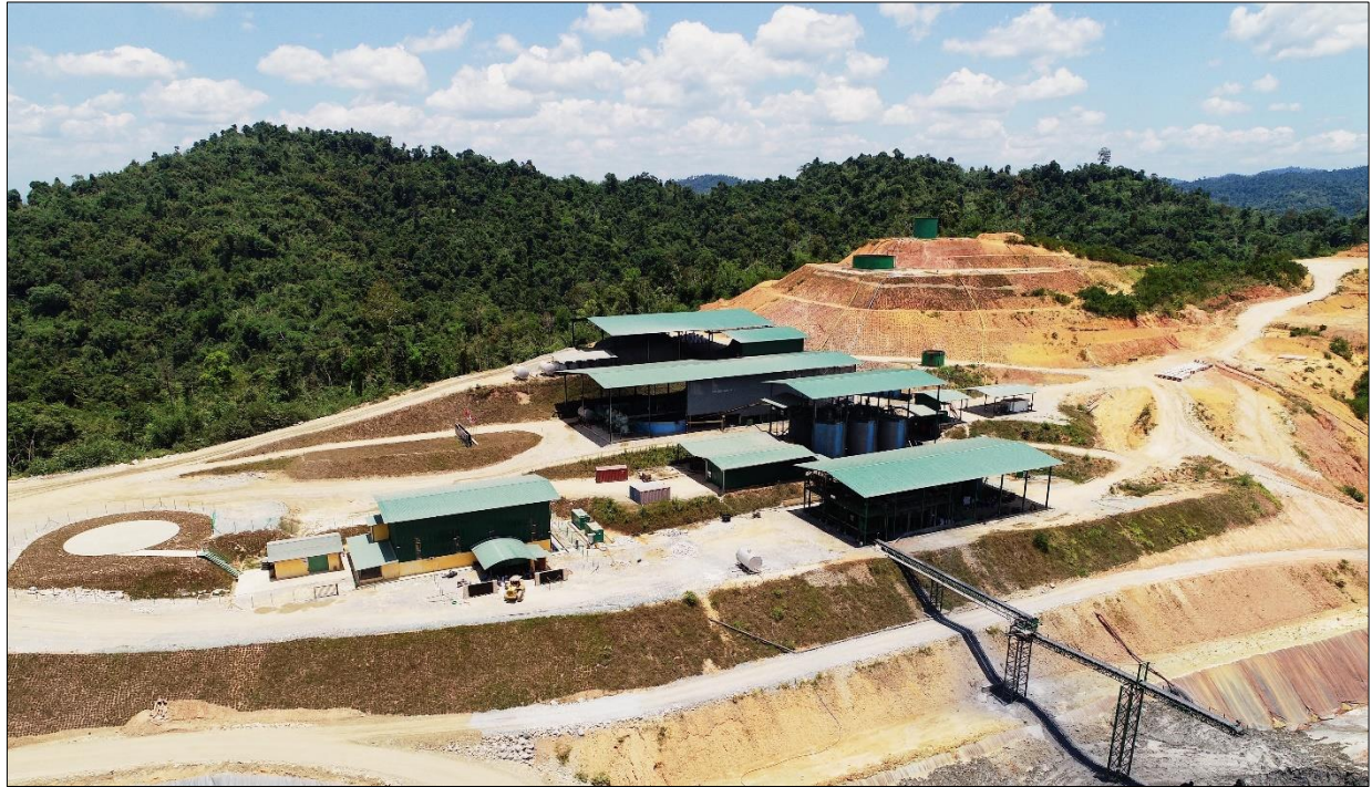
Figure 3.2 Sokor CIL plant and tailings facility – March 2019
