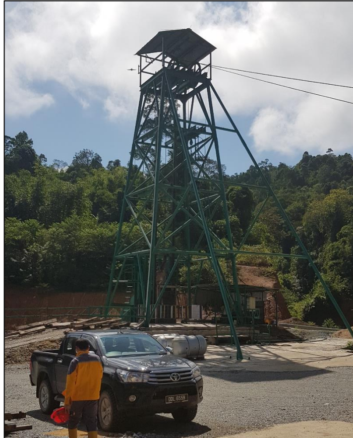
Figure 3.4 Ketubong shaft headframe – October 2019
