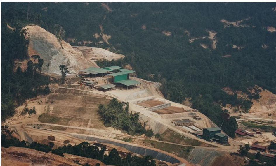
Aerial view of CNMC's newly upgraded Vat Leach Facility
