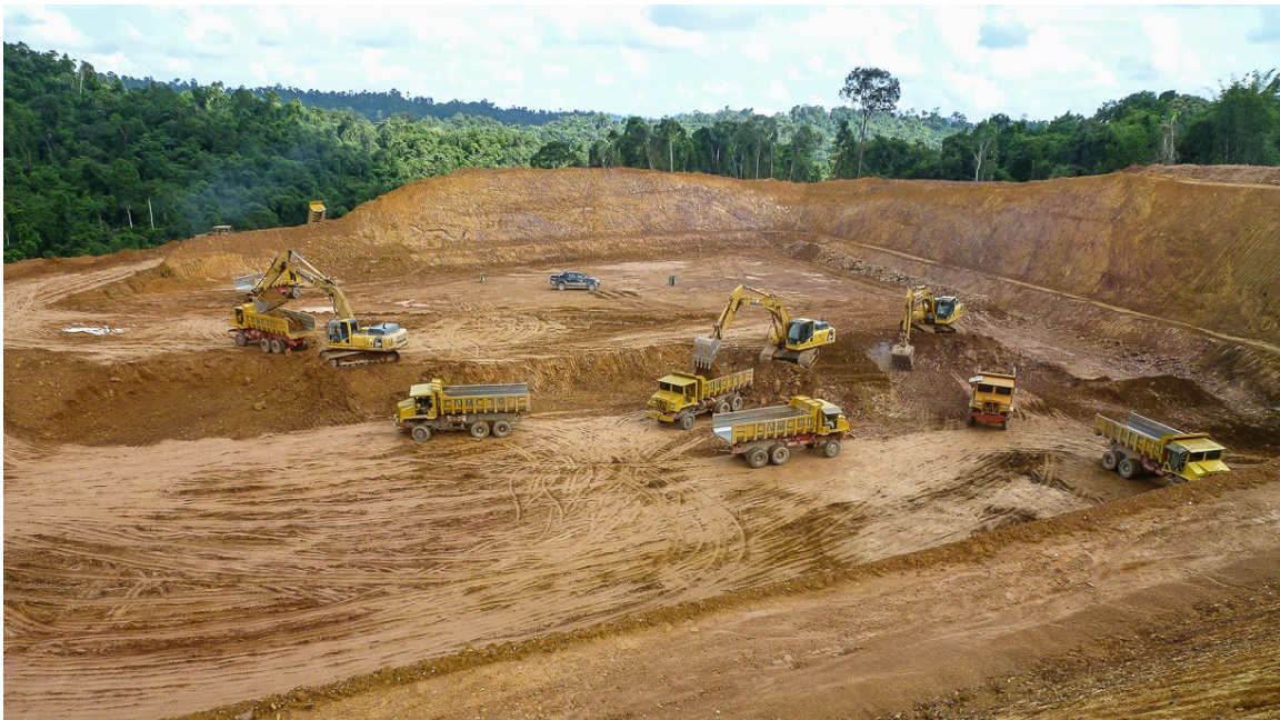
CNMC Photo: Construction of third leach yard in progress.
