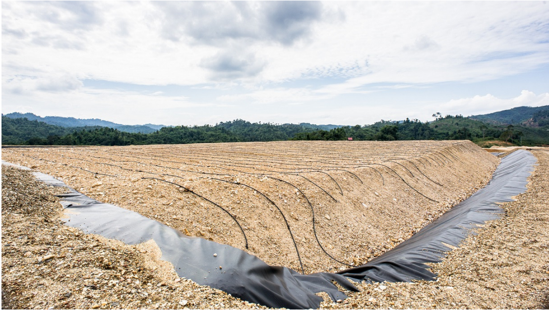
CNMC Photo: Completion of construction of second leach yard with approximately 140,000 tonnes of ore stacked.
