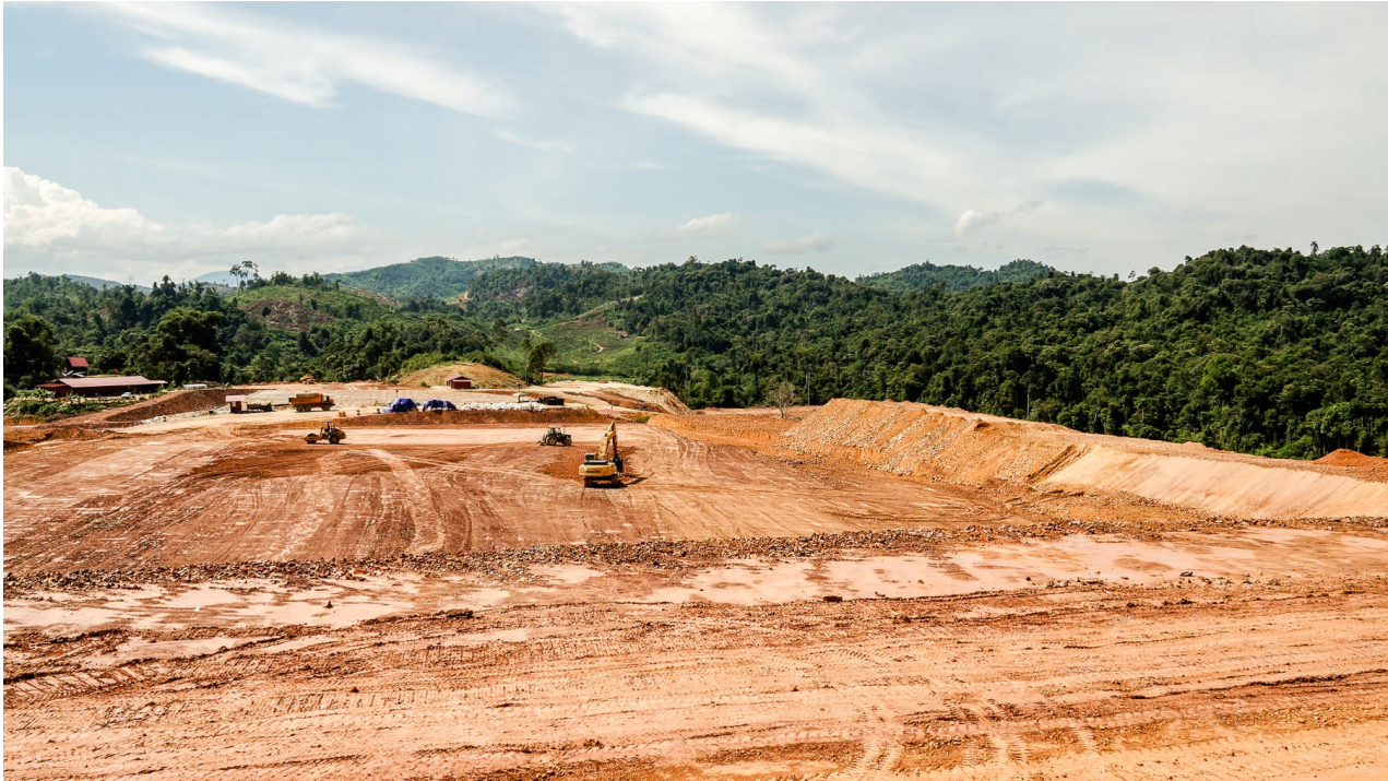
Second leach yard construction in progress as of 13 May 2013. PHOTO:CNMC
