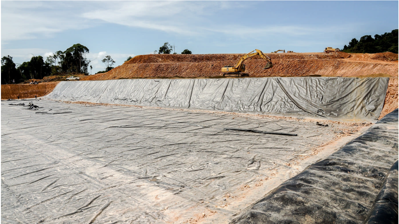
Second leach yard construction in progress as of 28 May 2013. PHOTO:CNMC
