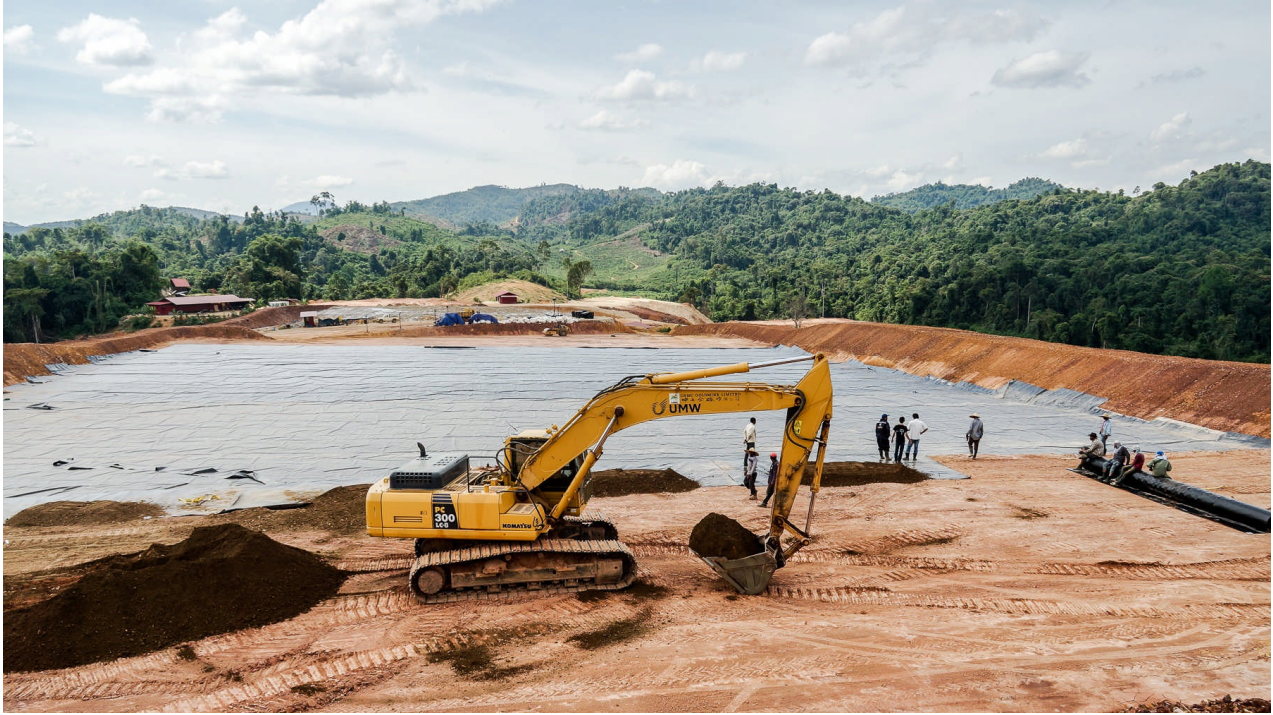
Second leach yard construction in progress as of 25 May 2013. PHOTO:CNMC
